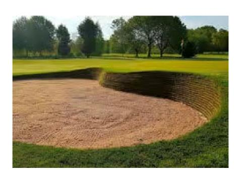
Our second generation synthetic bunker is constructed as a cantilever wall. This method builds upon our original concept by reducing waste whilst increasing structural ability.
